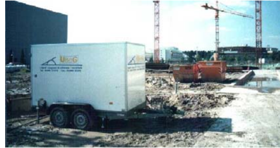
Figure 5: Test rig of UbeG GbR on site in Langen
