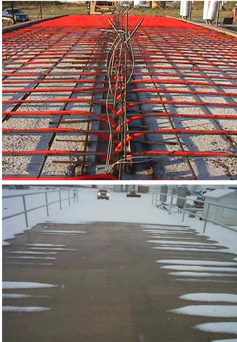
Figure 2 Geothermally Heated Bridge Deck at Oklahoma State University.
